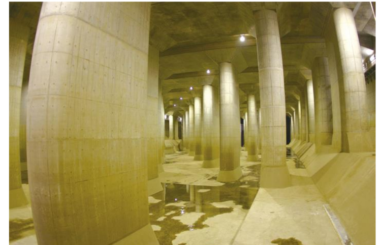
Metropolitan Area Outer Underground Discharge Channel Photo courtesy: Edogawa river office, MLIT
