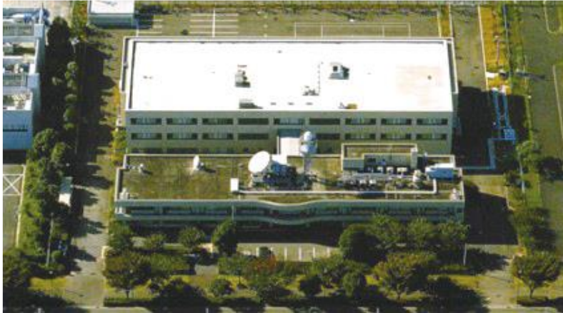
Disaster Management Headquarters Backup Facility
