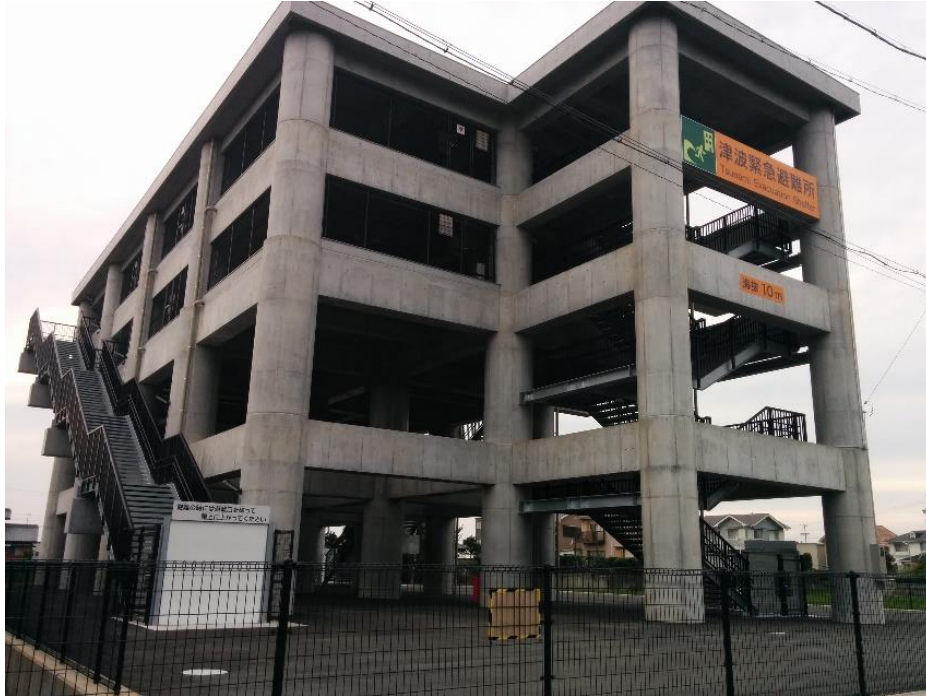
Tsunami Evacuation Tower (Ise City, Mie)
